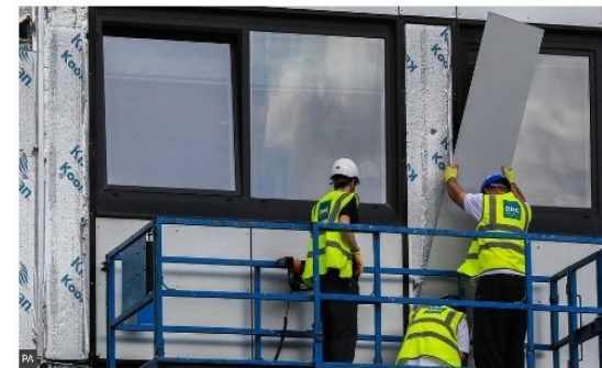
Cladding has been removed from numerous high-rise buildings following the Grenfell Tower fire
