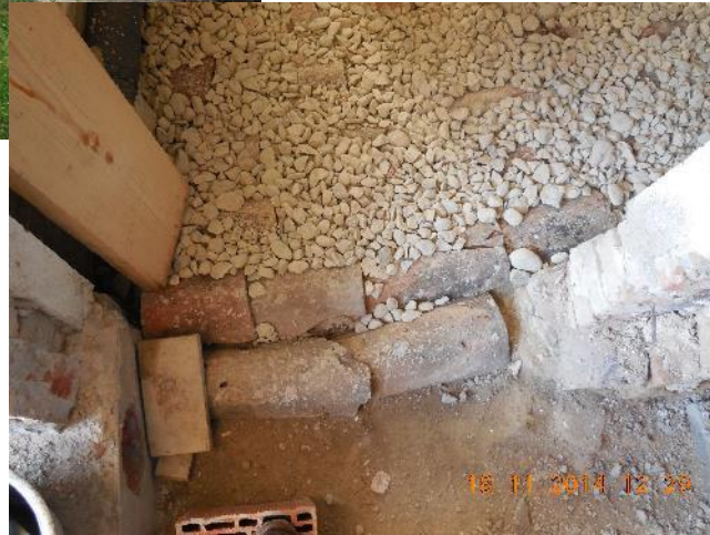
Tiles = crawl space
